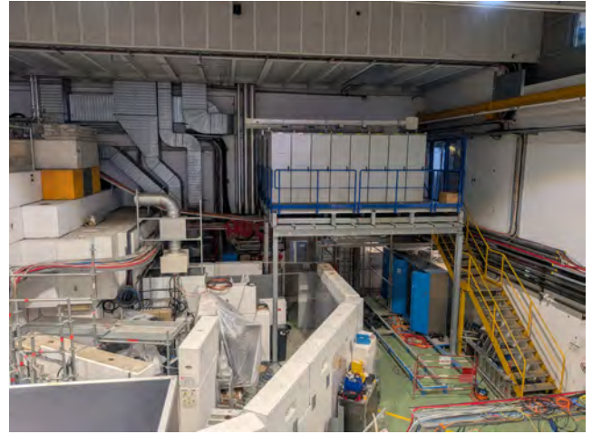
Figure 7: New platform in Building 170 for the installation of low-energy beamline electrostatic power-supply racks.
