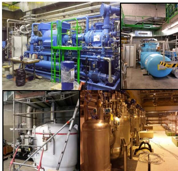
*Fig.1: Compressor station (top left); ex-ALEPH cold box in place (top right); Cryo Cold Line & Jumper Boxes installed in bldg. 170 (bottom).*
